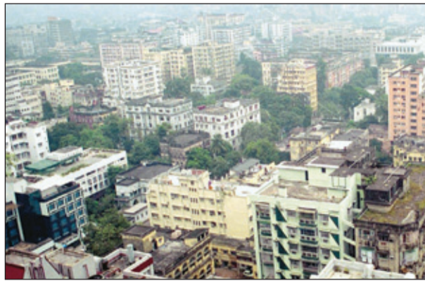
Highrise residents have blamed the administration for creating hurdles in the way of fire preparedness
